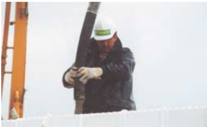
Figure 7: Pumping the concrete.
